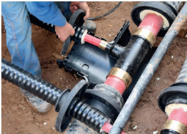
Abb. 4: The assembly process of the HeatClick Sleeve (Sleeve sealing ring)
