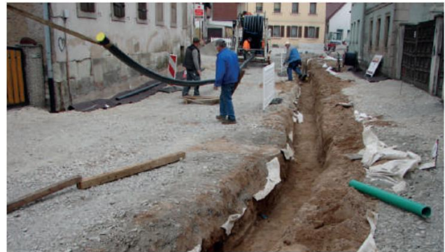
Abb. 30: open pipe trench with an uncoiling device
