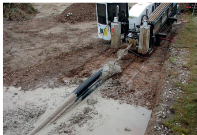
Abb. 29: flush drilling rig with pipes in the launch pit
