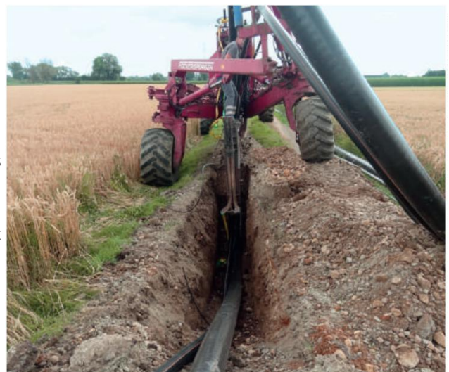
Abb. 27: Laying by plowing
