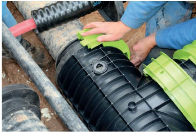
Abb. 3: The assembly process of the HeatClick Sleeve (locking ring)
