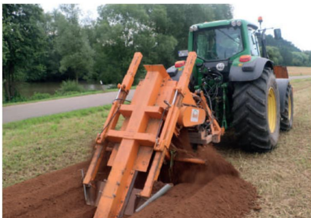
Abb. 28: Milling without installation box
