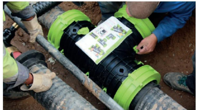
Abb. 5: The assembly process of the HeatClick Sleeve (clip)
