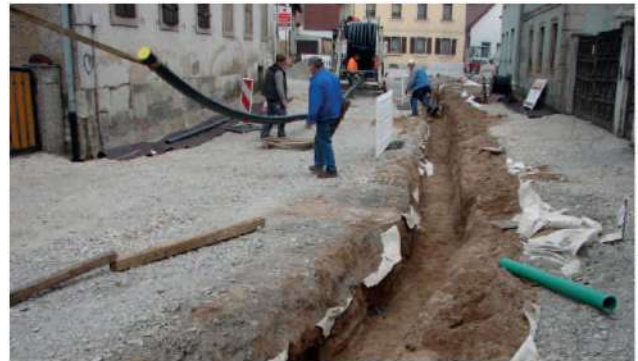
Abb. 30: open pipe trench with an uncoiling device
