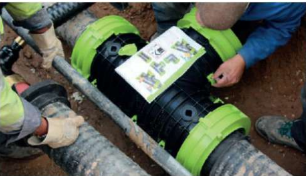
Abb. 5: The assembly process of the HeatClick Sleeve (clip)
