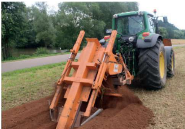
Abb. 28: Milling without installation box
