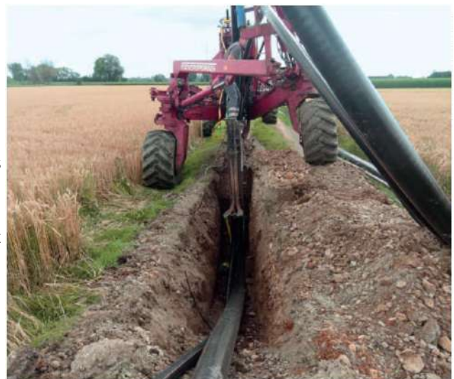
Abb. 27: Laying by plowing
