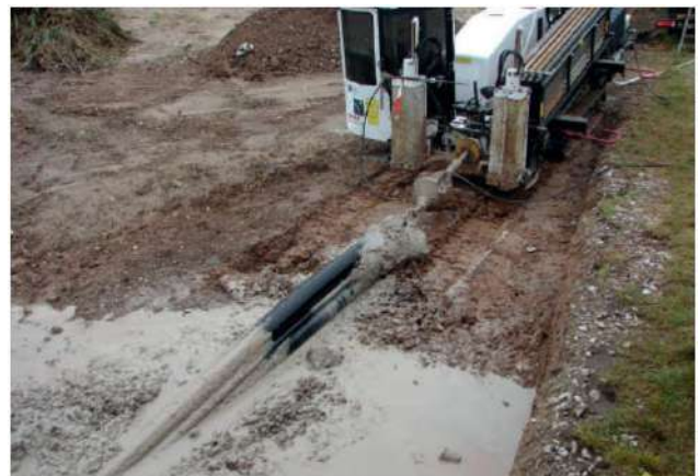
Abb. 29: flush drilling rig with pipes in the launch pit
