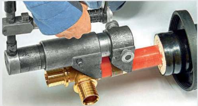
Pull the sliding sleeve over the body protector/ support. The connection is good if the medium pipe covers the last bar on the support body.
